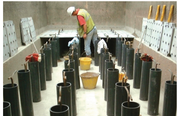
Column forms, cut to size and leveled
