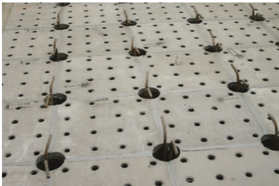
Panels sealed to column forms and abutting panel
