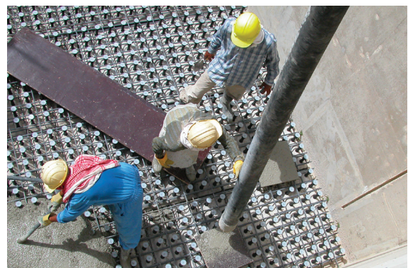
Pouring and vibration of concrete Trowel level to caps
