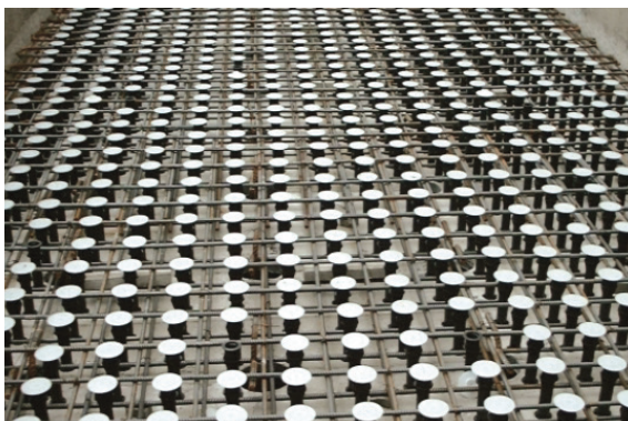
Installed threaded sleeves and protection caps
