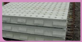
Precast Media Retention Slabs for Nozzle Deck
