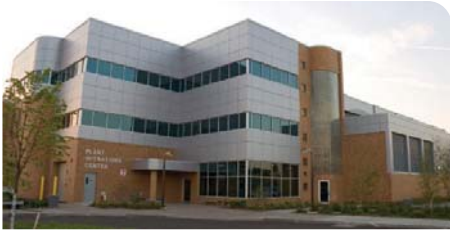
Syracuse, NY Onondaga County wastewater treatment plant
