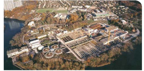
Geneva, Switzerland Aire wastewater treatment plant
