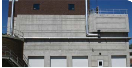
Kaukauna, WI Heart of Valley wastewater treatment facility
