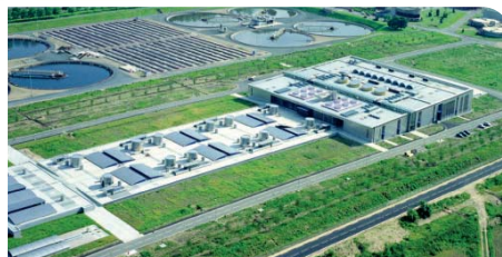
Paris, France Seine-Aval wastewater treatment plant
