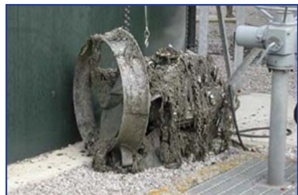
Typical ragged up submersible mixer, which has to be lifted out of the tank for cleaning
