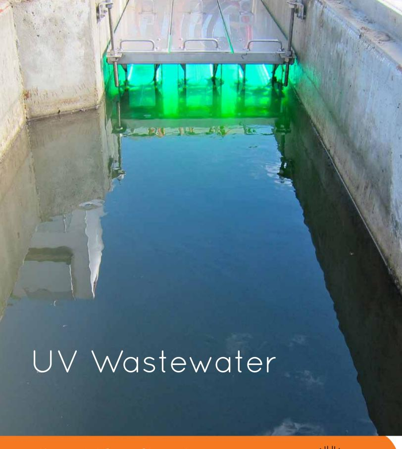
Horizontal Open Channel Ultraviolet Disinfection
