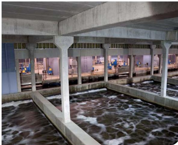
*Treated effluent at top of cells*
