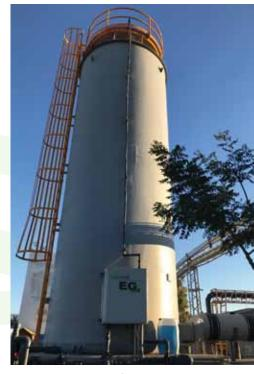
The EG-systems are designed for each application. Our EG-systems are designed with the appropriate Empty Bed Residence Time for long-term performance with extremely low operating costs.
