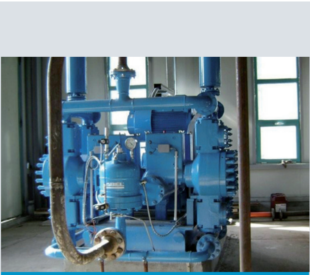
ABEL HMQ with reverse valves for transfer of fly ash with portions of coarse bottom ash
