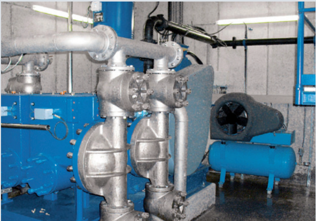
ABEL HMQ with stainless steel wet ends for transporting brine slurry
